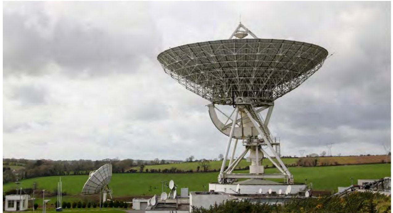
Figure 27: National Space Centre Ltd's 'Big Dish' received the first phase of remediation for preservation and re-purposing for a new future in Deep Space Communications © NSC Ltd.
